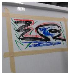
1. Apply a masking tape to avoid drip through.
